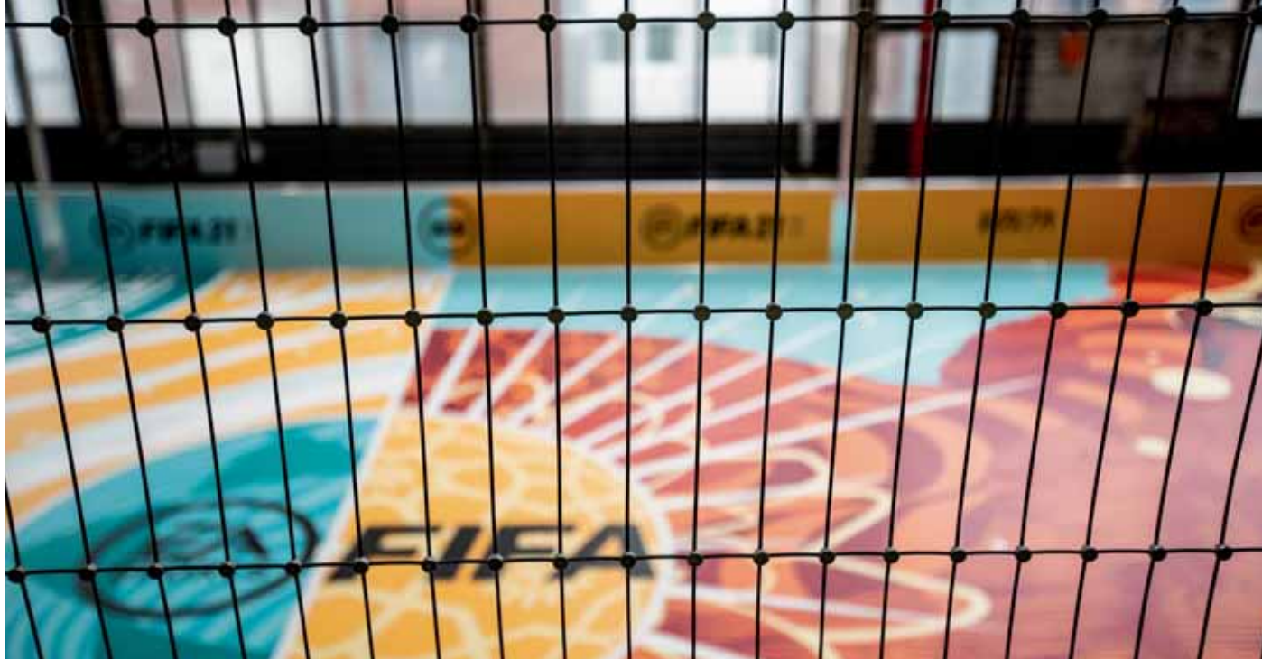
Anti-vandalism nets made of PA coated steel cable 1.8/2.5mm (see page 10.8). Made in collaboration with the company FUNTEC
