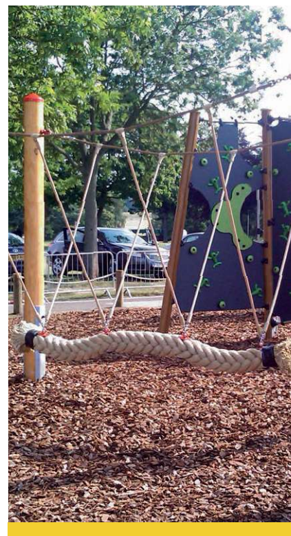
Design here with Douglas fir posts
